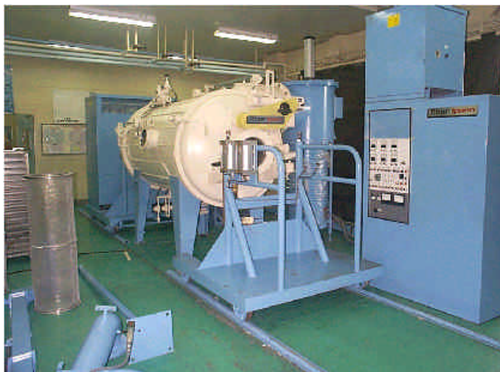
Figure 2. Barrel Coater Installation
